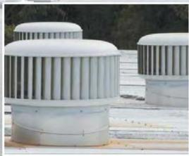
The Hurricane™ is a wind-driven roof exhaust fan. This natural ventilator is an alternative to traditional industrial ventilators that perform poorly and consume energy. Natural ventilation is proven to be effective and keep operating costs down.
