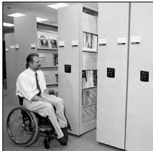
Figure 5. Unobstructed reach ranges can be applied to mobile storage. The controls must fall within a height range of 15–48 inches (380–1220 mm) from the floor.
