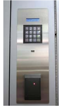
Touchpad interface with USB interface and protected LCD display
