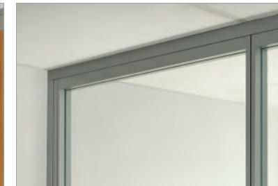
Traditional Crown stands slightly proud of the wall panel.
